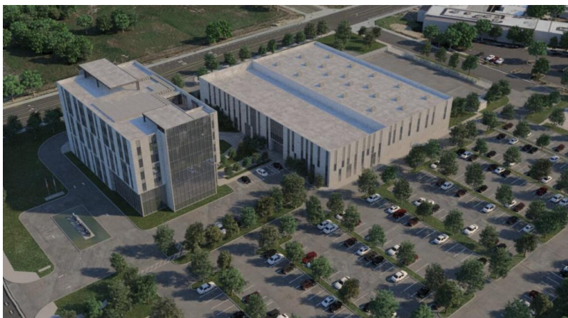
Advantech Campus – South Elevation
